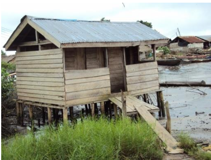
Plate 4.2o: An Over-hung Toilet in a Riverine Community in Bayelsa State
